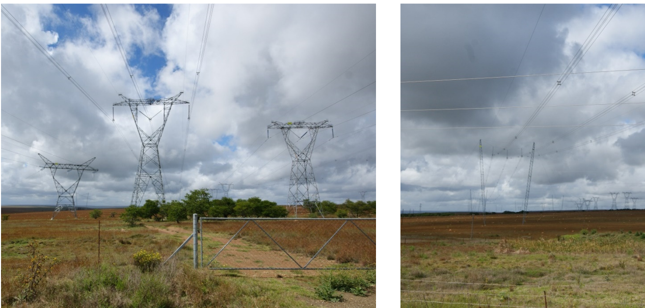
Figure 6: Examples of a self-supporting tower (left). Example of a cross-rope suspension tower (right).
